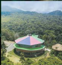
The Lillian Meighen Wright Centre, the landmark building of the York University EcoCampus. (Photo by Ofo Marin)
